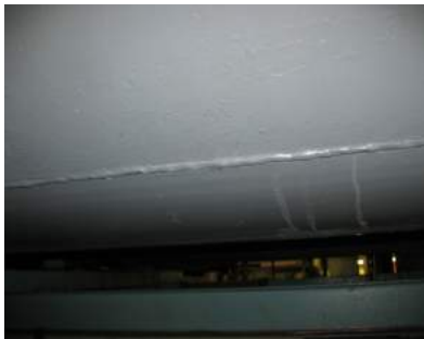
Expansion Tank - New Welded Bottom – Image 6
