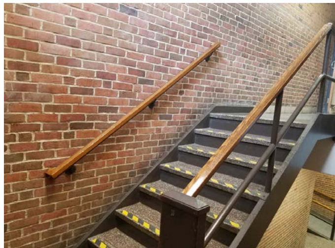
Handrails are noncircular, do not extend at the top and bottom and are interrupted by post. Stair has abrupt nosings.
