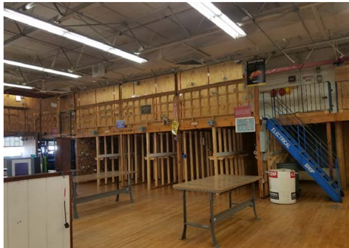
No accessible route to the upper level.
