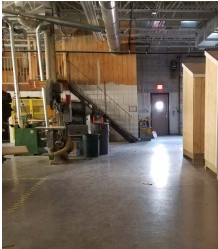
No accessible route to the upper level.
