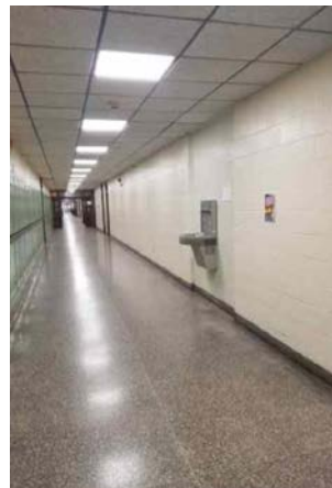
Protruding into the corridor more than 4 inches.
