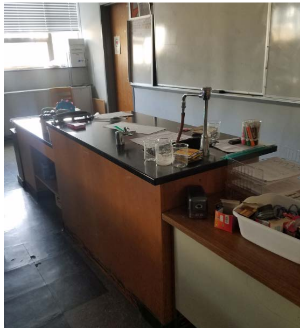
Non-accessible sink and counter space.
