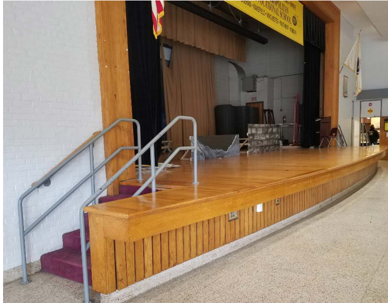
Stairs are the only way to access the stage.
