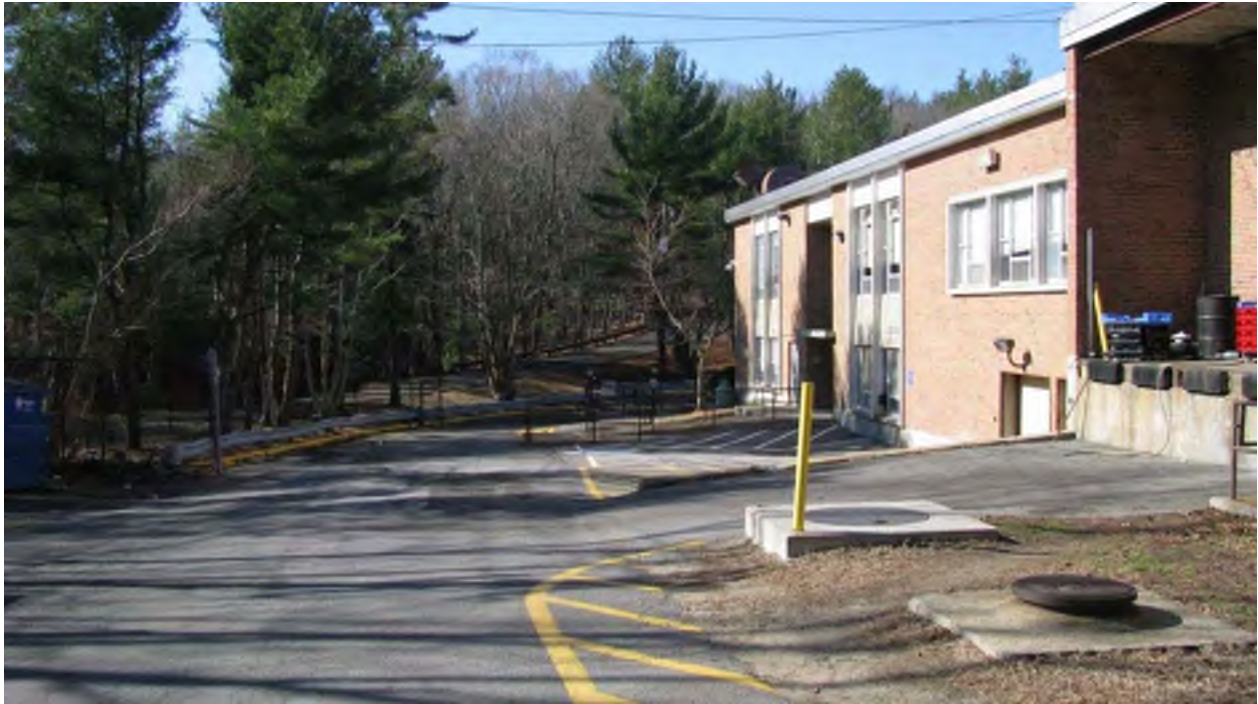
Photo 3. View looking south from the building's east side. The 20,000 gallon #4 fuel oil UST manhole covers are visible.
