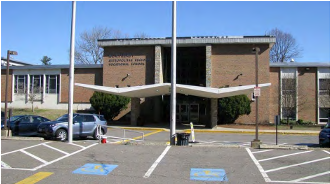
Photo 2. View of school front entrance from parking lot.
