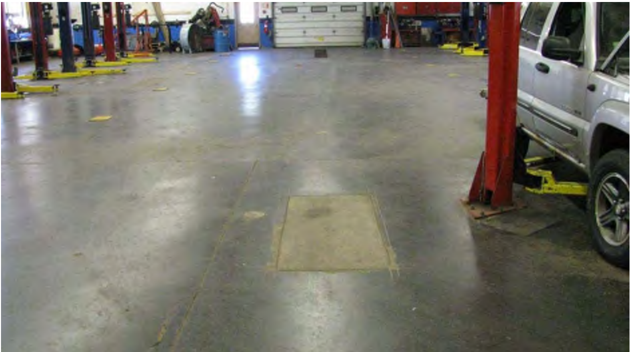
Photo 18. View of typical concrete floor patch indicating possible former hydraulic lifts.
