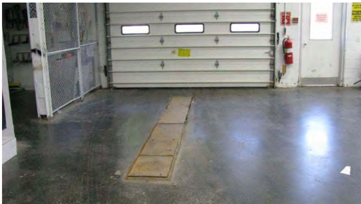
Photo 19. View in the Auto Body Shop of a former underground structure.
