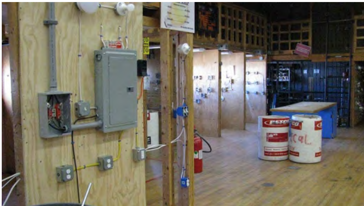
Photo 12. View of the Electrical Shop.
