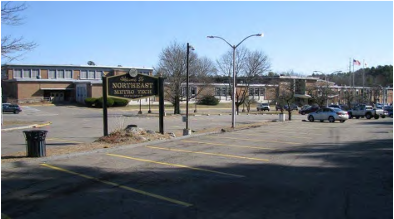
Photo 1. View of school building from front parking lot.
