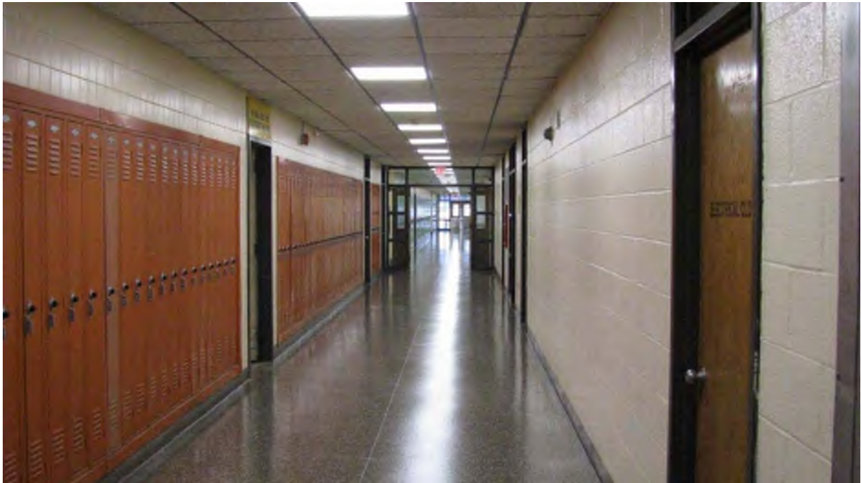
Photo 9. View of a typical hallway with tiled concrete floors, cinder block walls, and drop ceilings.
