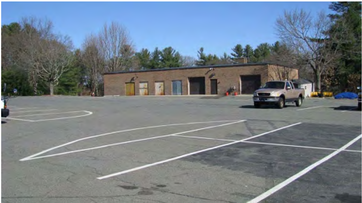
Photo 8. View of a maintenance building at the northwest corner.
