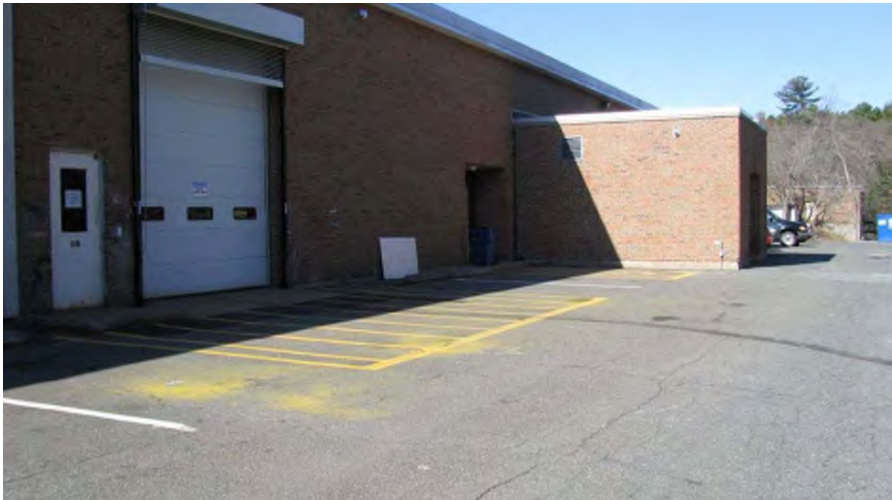
Photo 6. View of the northeast building corner and the Auto Body Shop bay door.
